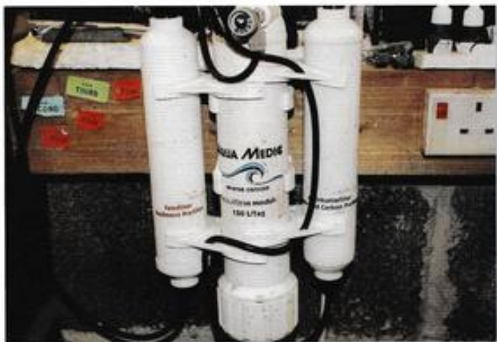
Since the water in their area is hard, an Aqua Medic RO unit is used to produce soft water to mix with tap water to create exactly the right conditions for each fish.
